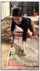
Spread the ¼ inch stone over the surface and into the joints. The ¼ inch stone is both bedding and filler for the joints. Add more stone the first 1-2 weeks as it settles into place.
