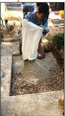
See cross section on page 1. 2 inches of 1/2 inch gravel topped with 2 inches of 1/4 inch gravel. Gravel should be clean and angular (no pea gravel or decomposed granite). Pack the gravel using boot compaction, a tamper, or flat board. Cover with plastic to keep clean when work stops.
