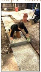
Using a notched board, screed the gravel 1.5 to 2 inches (whatever the thickness of the pavers or brick is) below the top of the edge restraints. This step is important to allow the top of the pavers to be level with the edge restraints and to each other. \*A level surface is very appealing with pavers.
