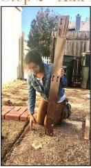
Restraints should be buried in the ground, level, and level to one another. Many different materials can be used (stone, concrete, laminated wood, and metal landscape borders, for example).
