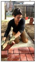
Some pavers have chamfers (ridges) on the side that form an open joint when layed. If they are bricks leave a ¼ inch joint between them on all sides. Make sure the surface of the pavers is level and place them neatly to form a nice, evenly aligned pattern.
