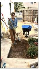
Excavate a minimum of 6 inches of soil making sure to maintain uniform depth along the edges and bottom. This depth, when filled with gravel, will capture about 1.5 inches of rain. Most rain events in central Texas are less than or equal to 1.5 inches.
